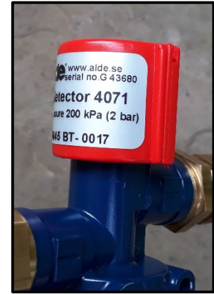
Figure 3. Post 2008 ALDE Leak Detector. Appendix D applies
