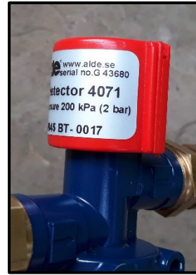
Figure 2. '4071' should be clearly visible on a label on the red test button.
