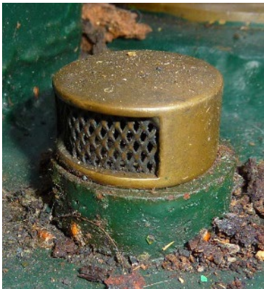
Water tank outlet with a mesh of less than 11 wires/cm
